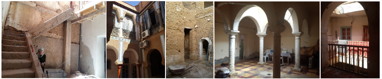
Fig. 2. Patios of the studied five houses in the Colonial Damier of Biskra.
